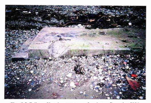
Plate 9.5: Failure of breakwater steps to foreshore, - December 2004.
