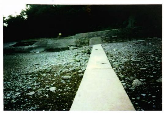
Plate 6.7: Concrete culvert for 1m diameter sea outfall.
