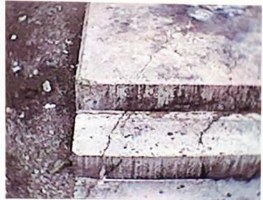
Plate 7.16: Tidal damage to steps (September 2002).
