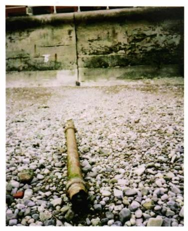
Plate 6.6: Exposed Victorian cast iron sewer
